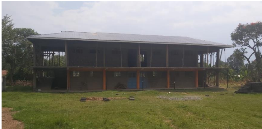
1 The Bishop Hannington Academy under construction
